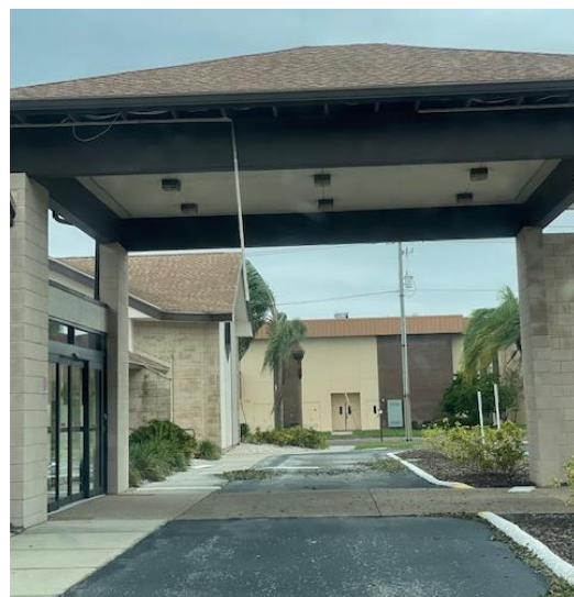
Soffit pieces missing under the portico.
